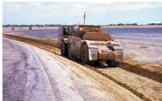
Photo 7.4. Excavation of a surface drain.
